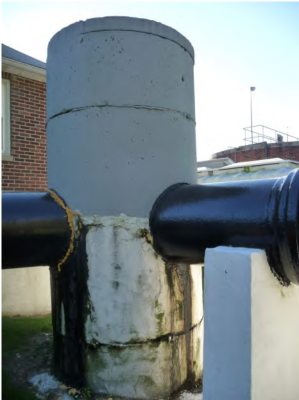
Picture 4: Manhole Downstream of Siphon Chamber
