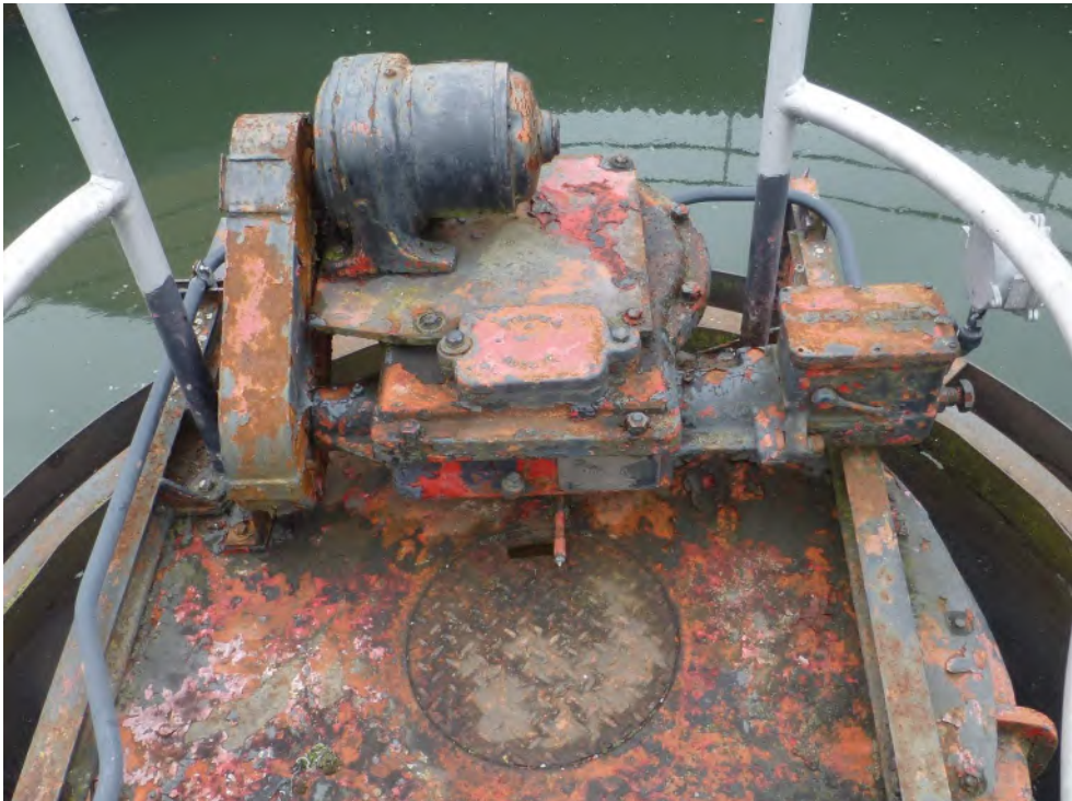
Picture 16: Drive Unit for Rake Arm
