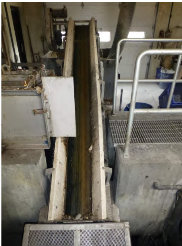
Picture 10: Conveyor cuts across channel
