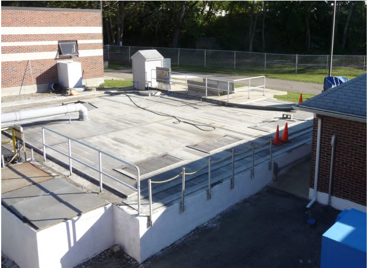
Picture 12: Pre-Aeration / Equalization Basin
