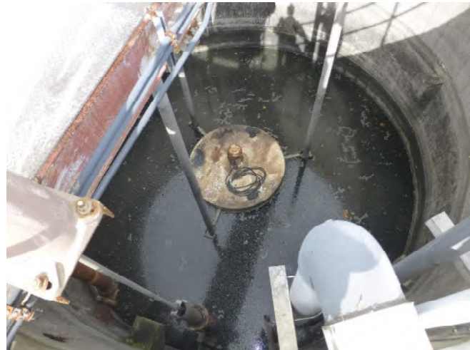
Picture 19: Small Sludge Holding Tank
