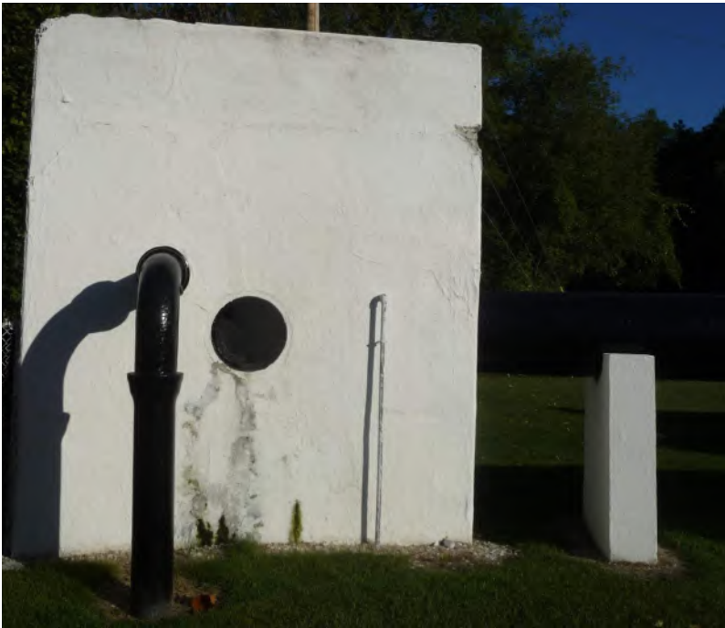
Picture 3: Siphon Chamber
