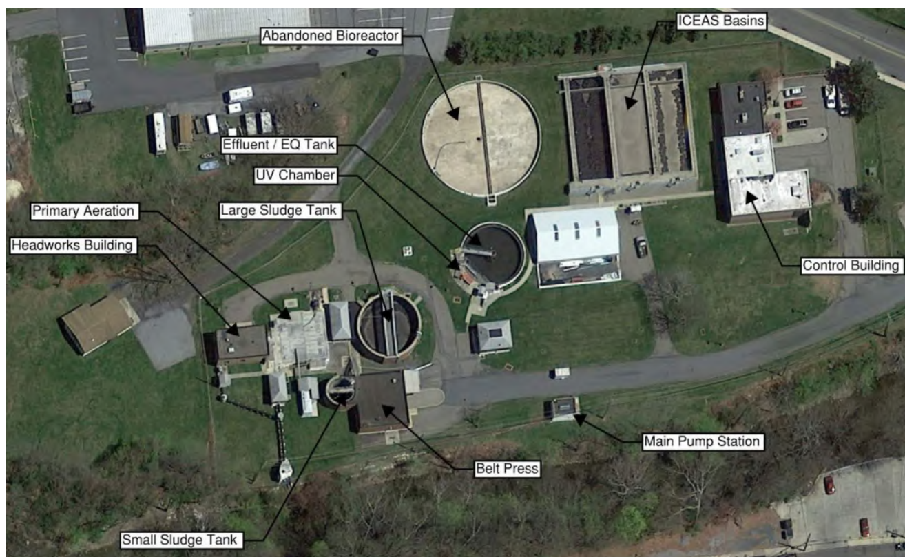
Figure 3: Overview of Equipment and Structures
