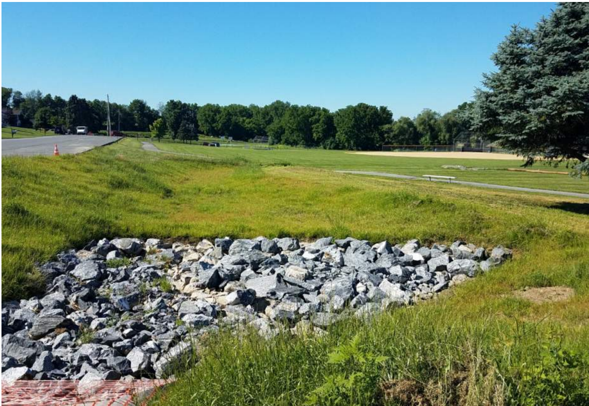
Photo (above): View of the vegetated swale for landscaping retrofit.
