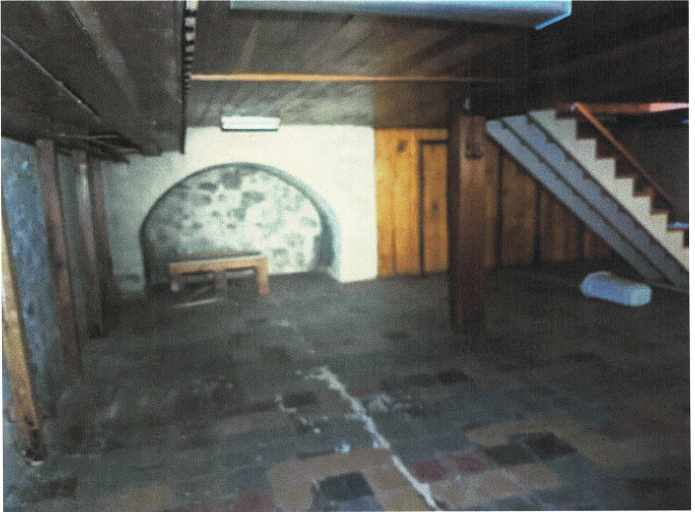
View of Asbestos Containing Floor Tile in Basement
